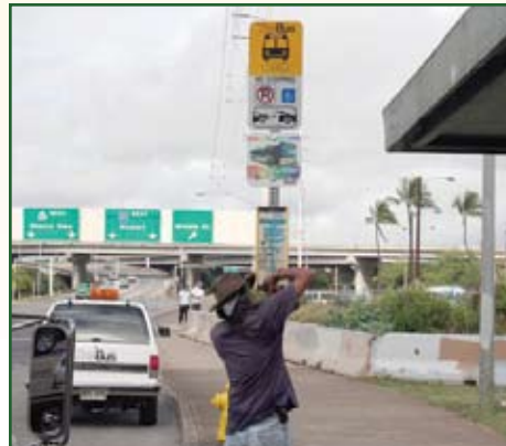
Photo Above: Tommy Balasbas repairing a bus stop sign.
